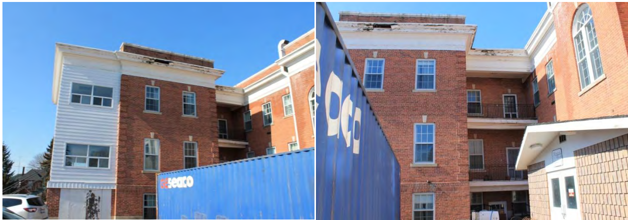
Figures 34 & 35: (left) View of east elevation of west wing, looking west (right)View of east elevation of west wing, looking west towards balconys/alcove (Source: MHBC, 2018)
