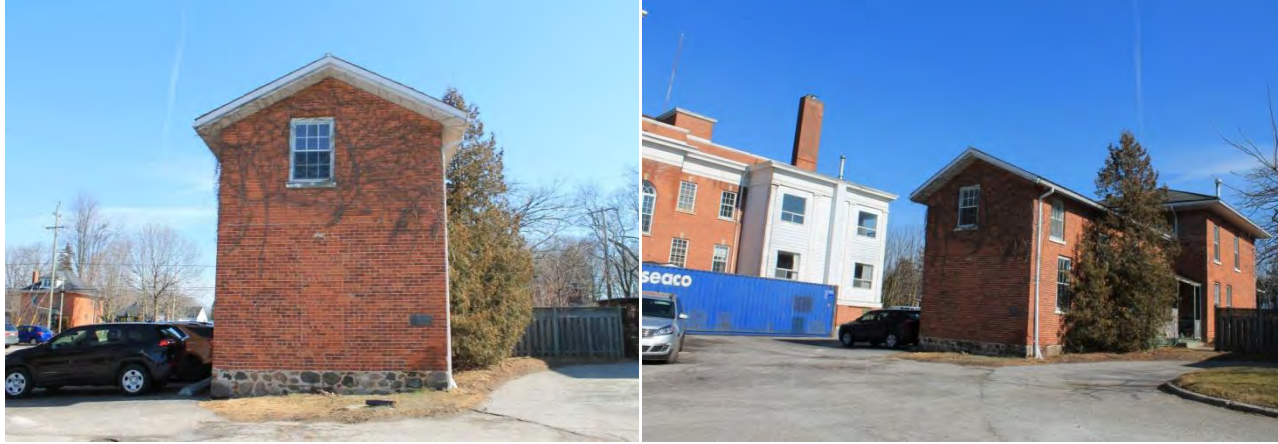
Figures 49 & 50: (left) View of west elevation, looking east towards second brick addition (right) View of south and west elevations, looking north-east (Source: MHBC, 2018)
