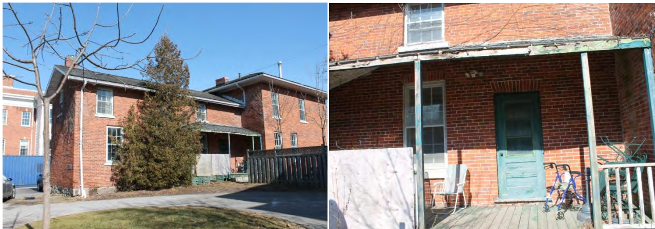
Figures 47 & 48: (left) View of south elevation, looking north-east (right) Detail view of wood frame portico at south elevation of first brick addition, looking north (Source: MHBC, 2018)
