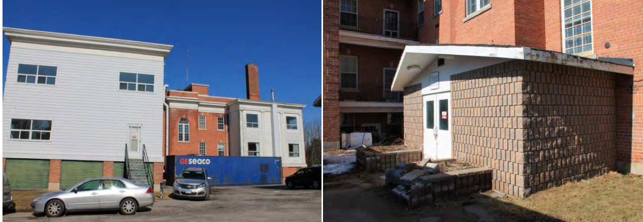
Figures 38 & 39: (left) View of south elevation looking north from parking lot (right) View 20 th century vestibule addition to south elevation of original portion of the building, looking north-west (Source: MHBC, 2018)
