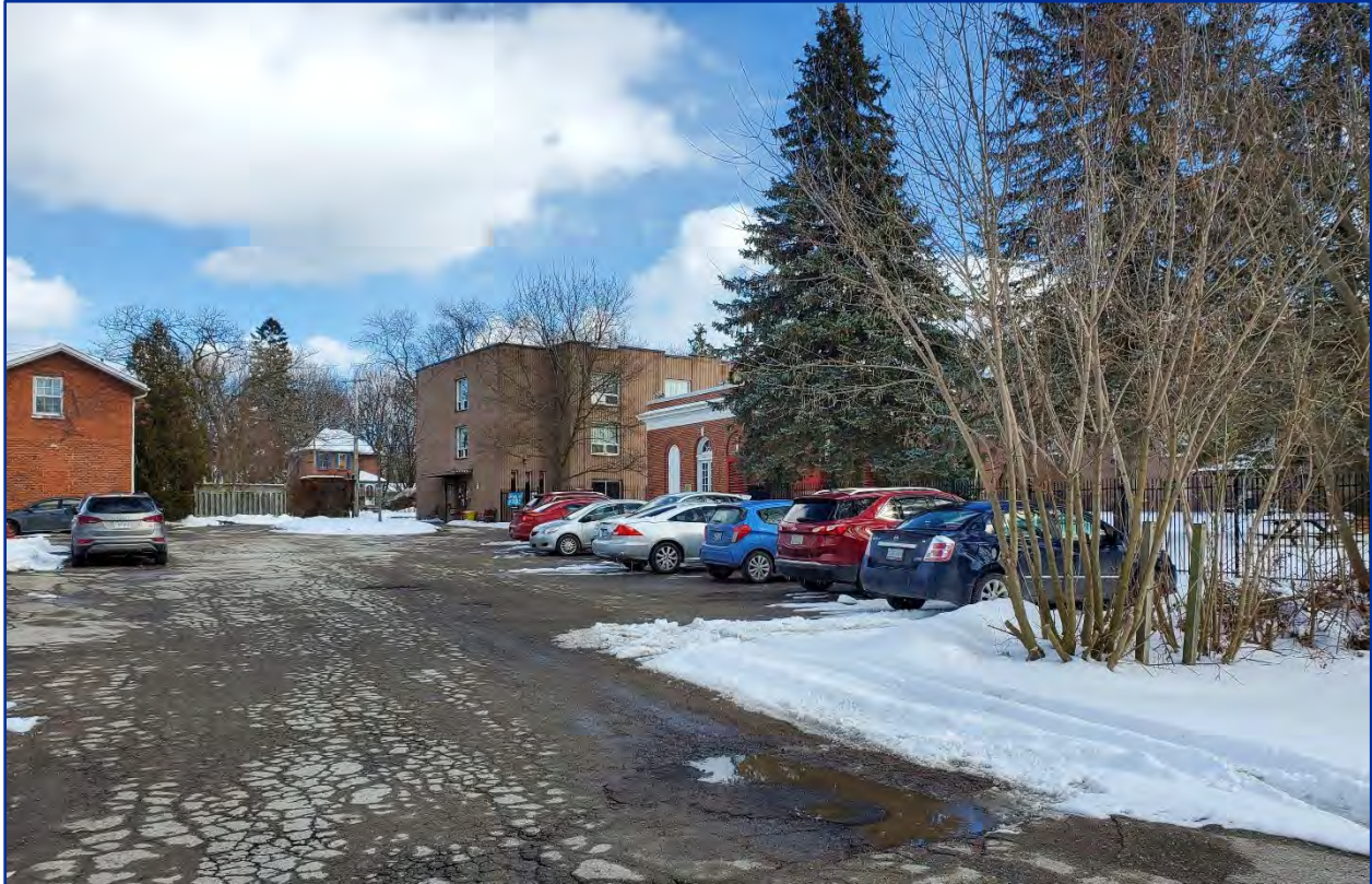
Figure 7 - View east of Power House
