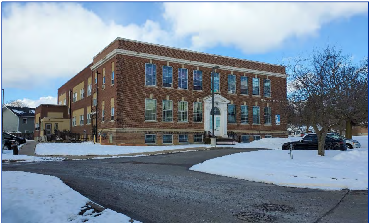
Figure 15: View north of former Dr. L.B. Powers School at 64 Ward Street
