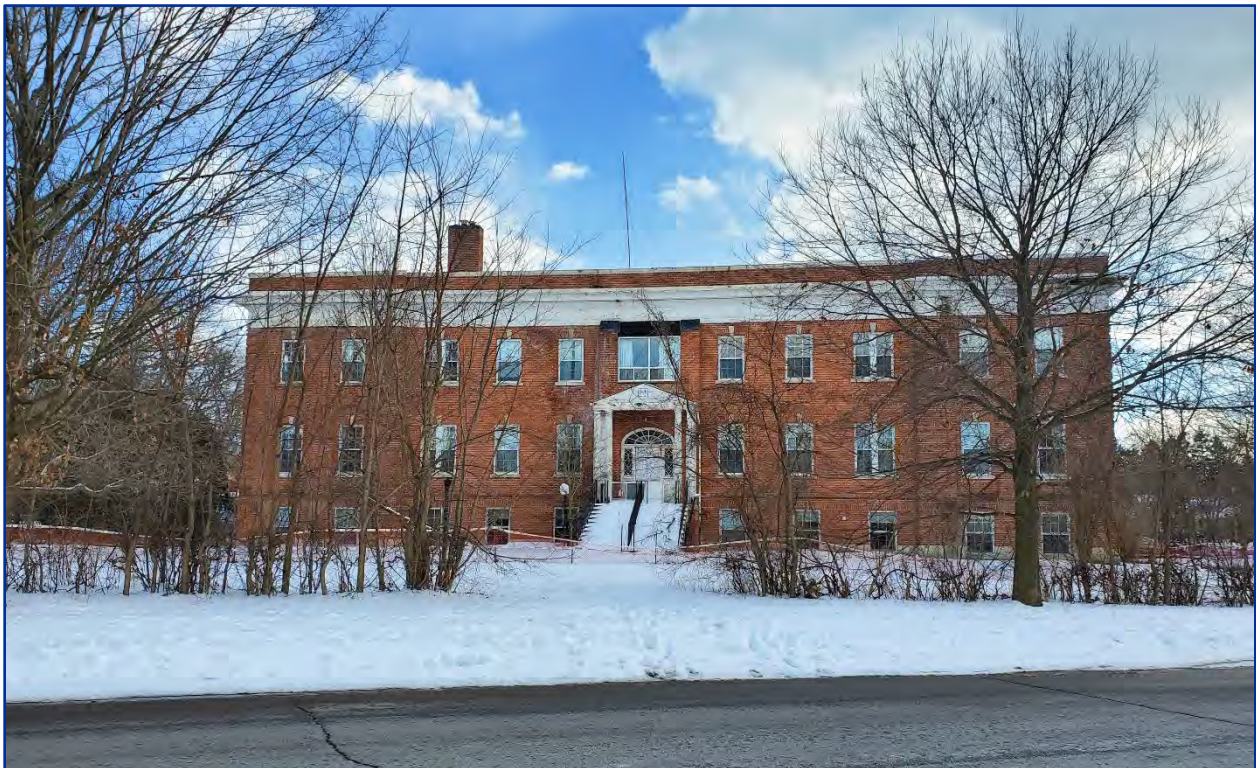
Figure 2: View south of north elevation
