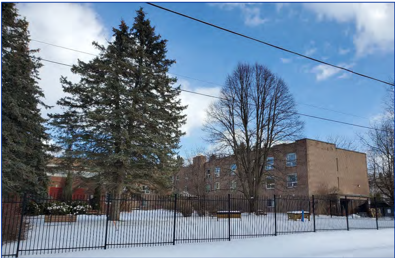
Figure 9: View southeast of Hope Terrace Care Facility
