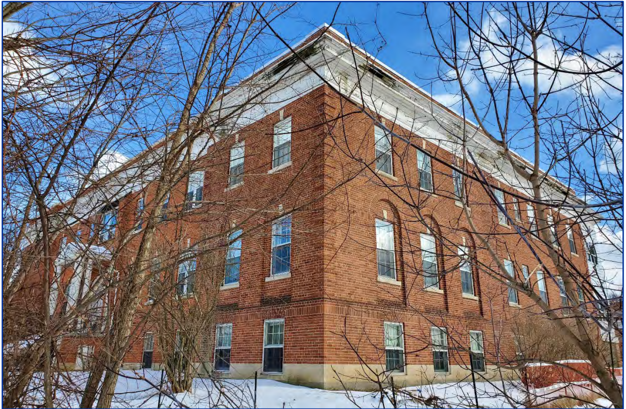
Figure 3: View southeast of northwest corner
