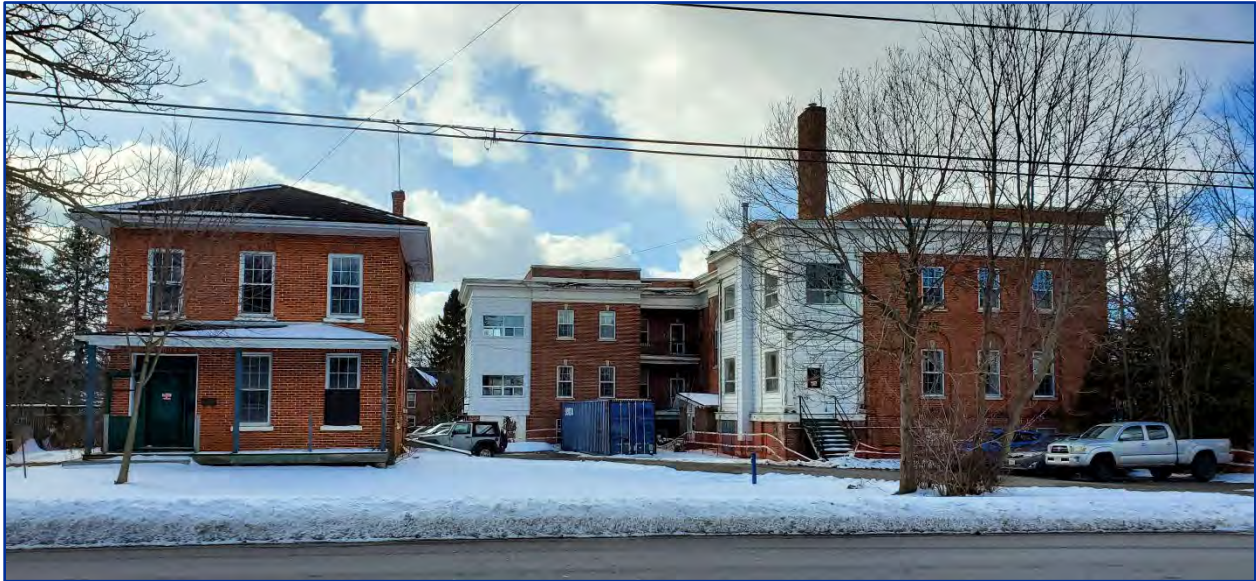
Figure 5: View west of east elevation and front of Cottage Hospital
