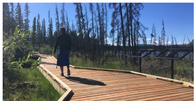
Boardwalk Accounting for Flooding
