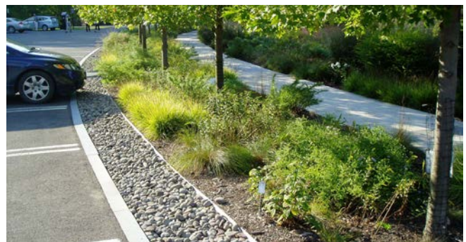
LID (Bioswales) incorporated into parking
