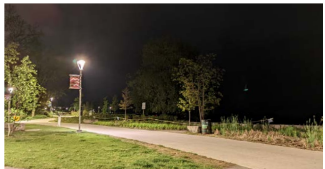
Lighting Fixtures for Pedestrians
