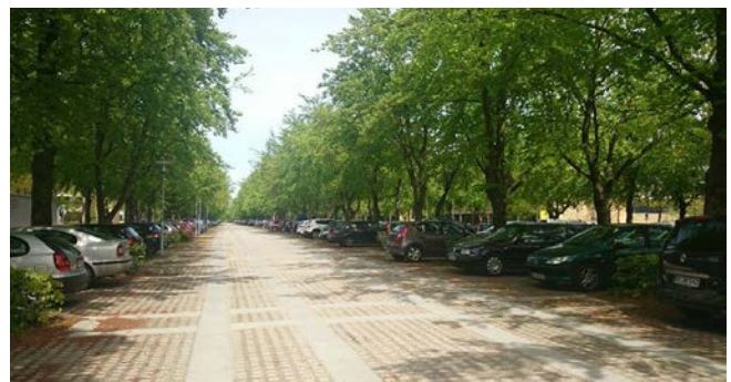
Permeable paving used for surface parking
