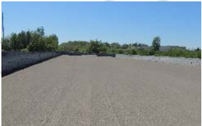
Sewage Treatment Plant Storage Cell
