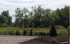
Sewage Treatment Plant TSS
