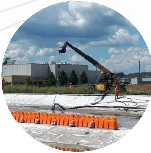
EQUALIZATION POND CLEANOUT
