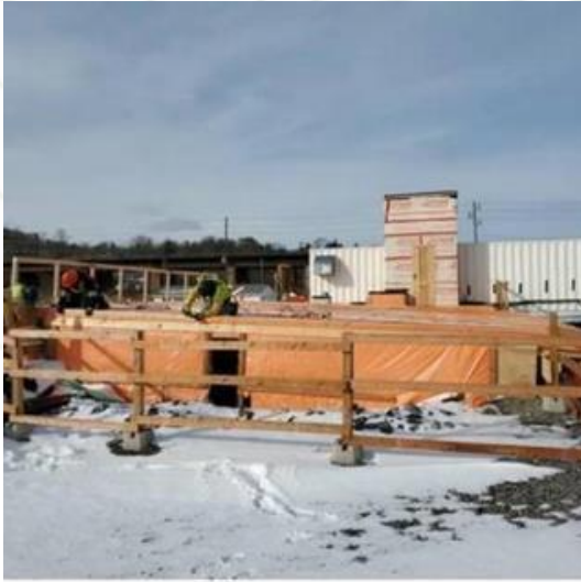
Winterization of water treatment system components
