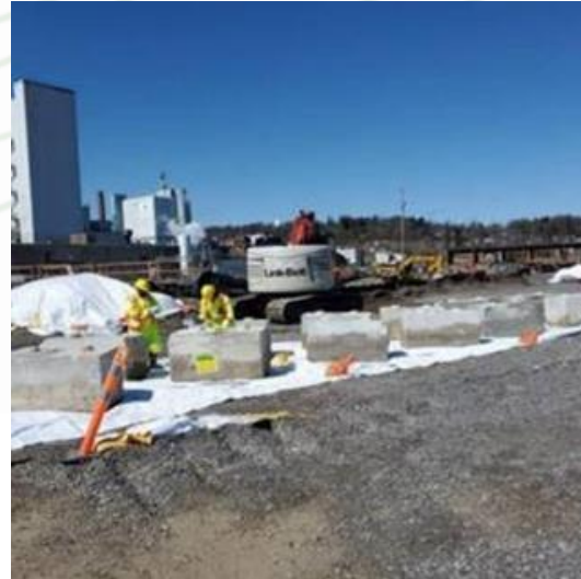
Removal of debris from dewatering area and reconstruction of sediment dewatering area for mechanically dredged sediments
