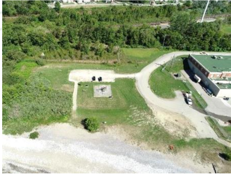
Waterworks West Expected to start 2022
