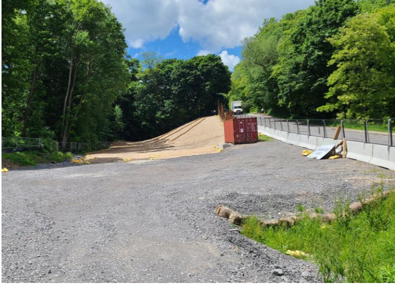
Strachan Street Ravine Restoration underway
