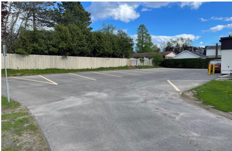
Figure 21: Rear parking area at Fire Station 1.
