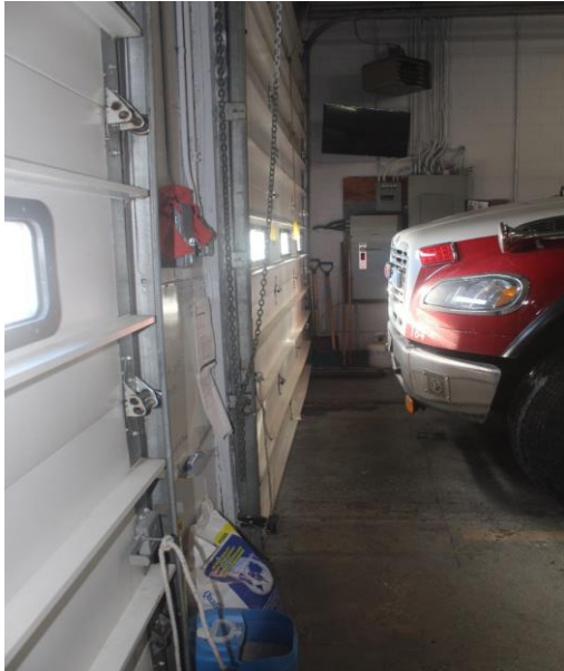
Figure 25: Front view of apparatus placement at Fire Station 2.
