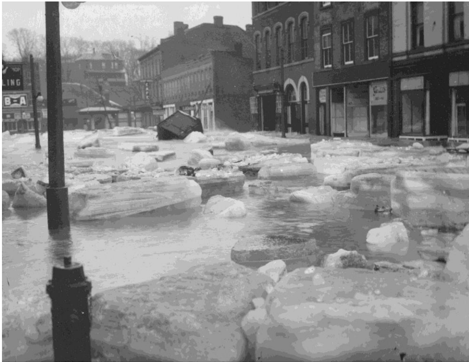
Figure 5: Flooding in downtown Port Hope.
