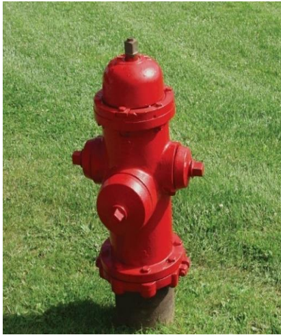
Figure 42: Picture of private hydrant.
