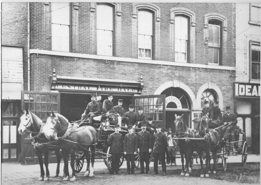
Figure 2: Exterior of the Central Fire Station.
