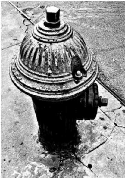
Figure 3: Fire hydrant in the downtown area.
