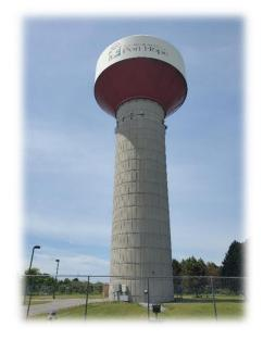
The **Fox Road elevated Tower** provides off-site storage tank that can hold up to 3,000 m3 of water.
