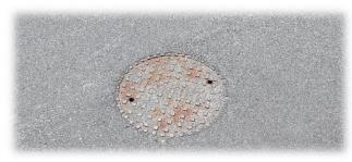
The purpose of a **storm**Maintenance Hole is to allow for a human access point at certain intervals of a storm drainage system for inspection and maintenance purposes.
