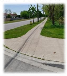
Being a surfaced walkway, separated from the roadway, usually of concrete and following the existing ground surface (not at permanent grade), **sidewalks** are found in certain areas within the urban boundary.
