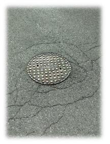
The purpose of a **Wastewater Maintenance Hole** is to allow for a human access point at certain intervals of a wastewater drainage system for inspection and maintenance purposes.
