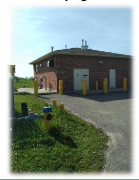
The AON Wastewater Pumping Station (WWPS) is a wet well/dry well style station constructed in 2005/2006 and located at 435 Lakeshore Road ±200 m south of Lakeshore Road. The catchment area serviced by the AON WWPS generally encompasses most lands west of Toronto Road
