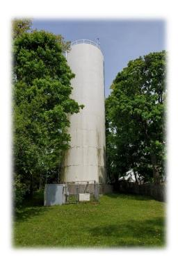
The **Dorset Street Standpipe** provides off-site storage facility in Zone 1 includes a standpipe with a rated capacity of 1,080 m<sup>3</sup>.
