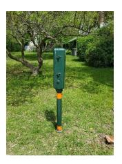
sampling stations give operators unrestricted access to sample sites, provide a dedicated tap for sample retrieval with no outside crosscontamination, and allow for samples to be taken directly from the water main.
