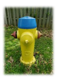
A hydrant is a visible fixture placed outside a building, parking area, industrial area, or roadside that is connected to the municipal or a private water service network. They are used for flushing the mainline; creating a scouring action to clean the line. Fire hydrants are designed to instantly provide the water required by fire fighters to extinguish a fire.
