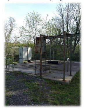
The Hope Street Wastewater Pumping Station (WWPS) is the smallest of the Municipality's three (3) pumping stations. Constructed in 1987/1988 the Hope Street WWPS is a submersible (wet well) style station located at 305 Hope Street North
