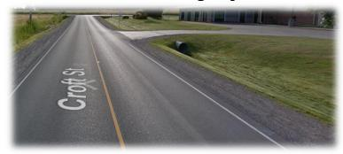
Flows that exceed the capacity of the storm sewers are conveyed along the ground surface (i.e. "overland"). The overland system makes up what is called the "major" **drainage system** since it conveys flows in excess of the minor system during larger magnitude, infrequent storm events. This system is made of swales and ditches with minor culverts.
