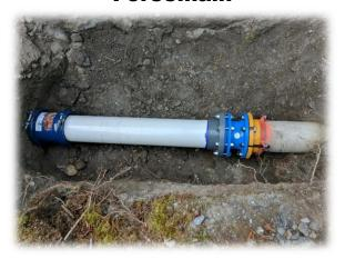
A **force main** is a pressurized sewer pipe that conveys wastewater under pressure from the discharge side of the pump. Force mains are used where gravity is not enough to move sewage or stormwater runoff through a sewer line
