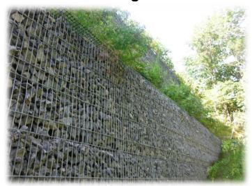
Retaining walls are relatively rigid walls used for supporting soil laterally so that it can be retained at different levels on the two sides
