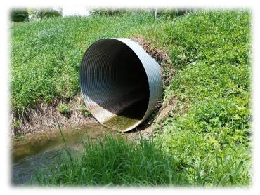
**Culverts** are a buried structure which carries a road or footpath while allowing stormwater to pass through.
