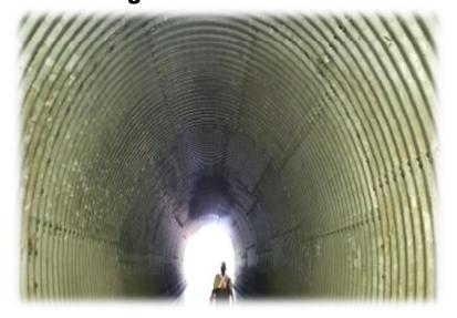
Large Diameter Culverts are a buried structure which carries a road or footpath allowing water to traverse it's natural path.
