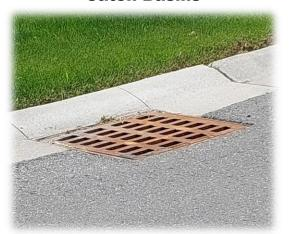
A **catch basin** is, in other words, a storm drain. They are used to redirect water to prevent flooding and are common on public streets. Catch basins collect rainwater or melted snow and transport it to an outfall reservoir.
