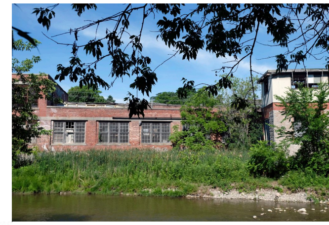
1902, East elevation overlooking river, 1 storey brick walls with concrete banding and wall cap, expressed pilasters, 6 part multi lite windows in 5 window bays with concrete lintels and sills
