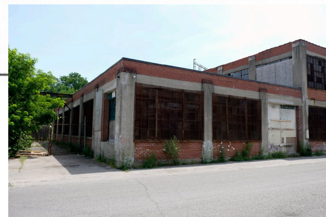
1935, 1 storey brick walls with expressed concrete pilasters with stepped brick capitals, full width window openings with concrete lintels and sills, large multi lite windows. North Elevation returning to east elevation with same attributes
