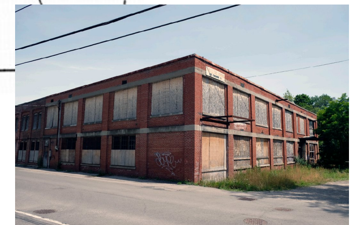
West elevation, 2 storey brick walls with concrete banding and wall cap, expressed pilasters, multi lite windows in 5 window bays
