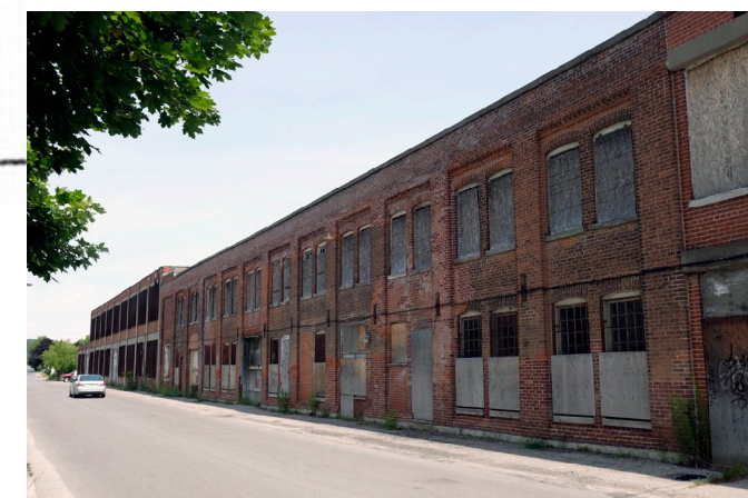
1900, 2 storey brick walls expressed pilasters denticulated step below parapet forming pilaster bays, paired ground and second floor windows with brick arched openings ( encourage restoration of altered ground floor openings)
