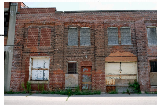
1889, 2 storey brick walls expressed pilasters, paired second floor windows with brick arched openings (ground floor altered several times, encourage some restoration at ground floor)
