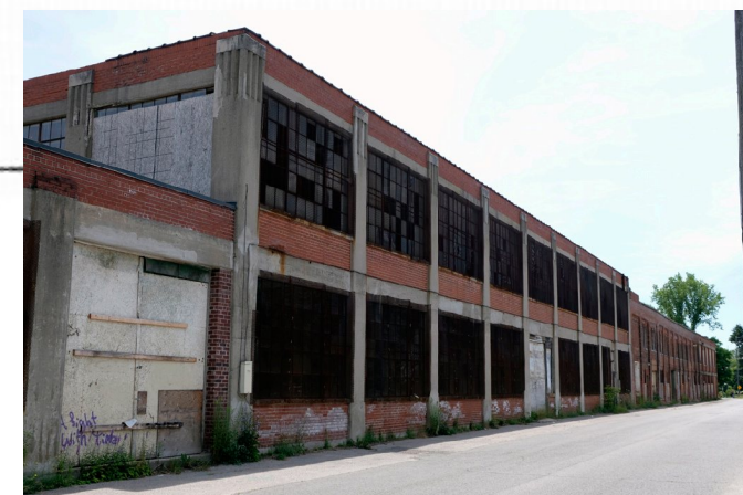
1935, 2 storey brick walls with expressed concrete pilasters with decorative Deco capitals, full width window openings at ground and second floor with concrete lintels and sills, large multi lite windows. North Elevation returning above #16 with same attributes
