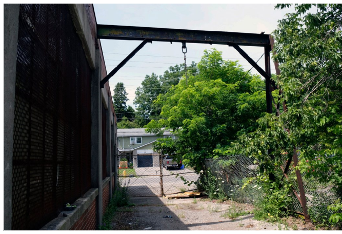
Exterior steel hoist structure, preserve on site
