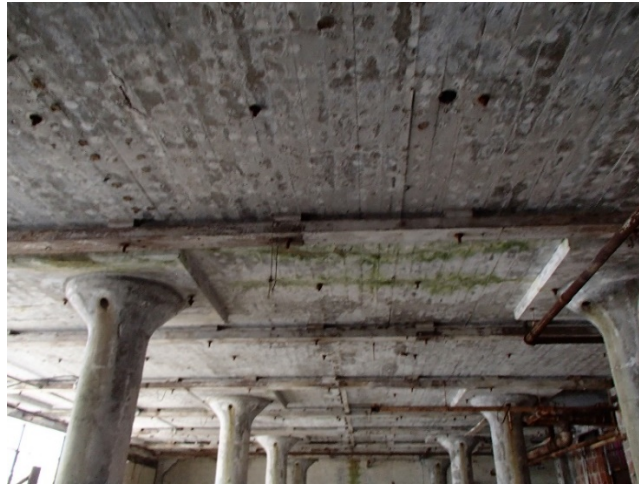
Photo 7: Ground Floor Level Looking up at Underside of 2 nd Floor – Block #5
